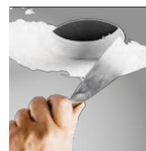
skimmed into plasterboard ceiling (trimless)
