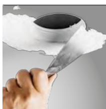
skimmed into plasterboard ceiling (trimless)
