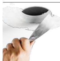
skimmed into plaster- board ceiling (trimless)
