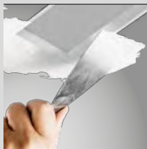
skimmed into plasterboard ceiling
