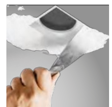
skimmed into plasterboard ceiling (trimless)
