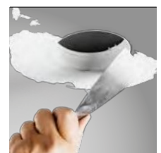
skimmed into plasterboard ceiling (trimless)
