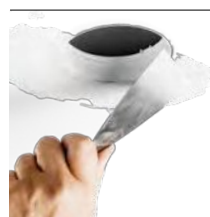
skimmed into plasterboard ceiling (trimless)
