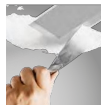
skimmed into plasterboard ceiling (trimless)
