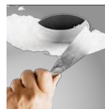
skimmed into plasterboard ceiling (trimless)
