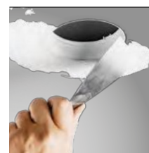
skimmed into plasterboard ceiling (trimless)
