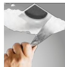
skimmed into plasterboard ceiling (trimless)
