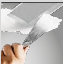
skimmed into plasterboard ceiling
