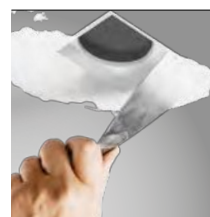
skimmed into plasterboard ceiling (trimless)
