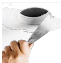
skimmed into plaster- board ceiling (trimless)
