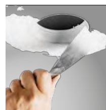
skimmed into plasterboard ceiling (trimless)
