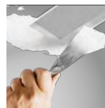
skimmed into plasterboard ceiling (trimless)
