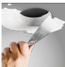
skimmed into plasterboard ceiling (trimless)
