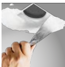
skimmed into plasterboard ceiling (trimless)
