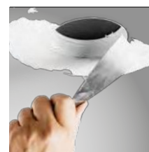
skimmed into plasterboard ceiling (trimless)
