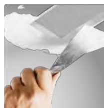
skimmed into plaster- board ceiling (trimless)
